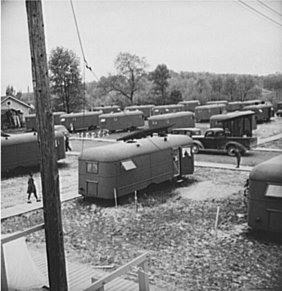
Figure 3. An April 1942 general view of a trailer camp on the future site of the Carver Apartments. The federal government established the camp for African Americans displaced by the construction of the Pentagon.
