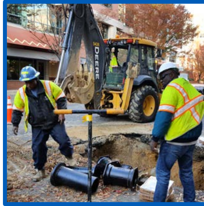
STATE OF GOOD REPAIR
