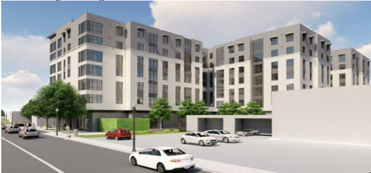
Figure 2--View from Southeast
