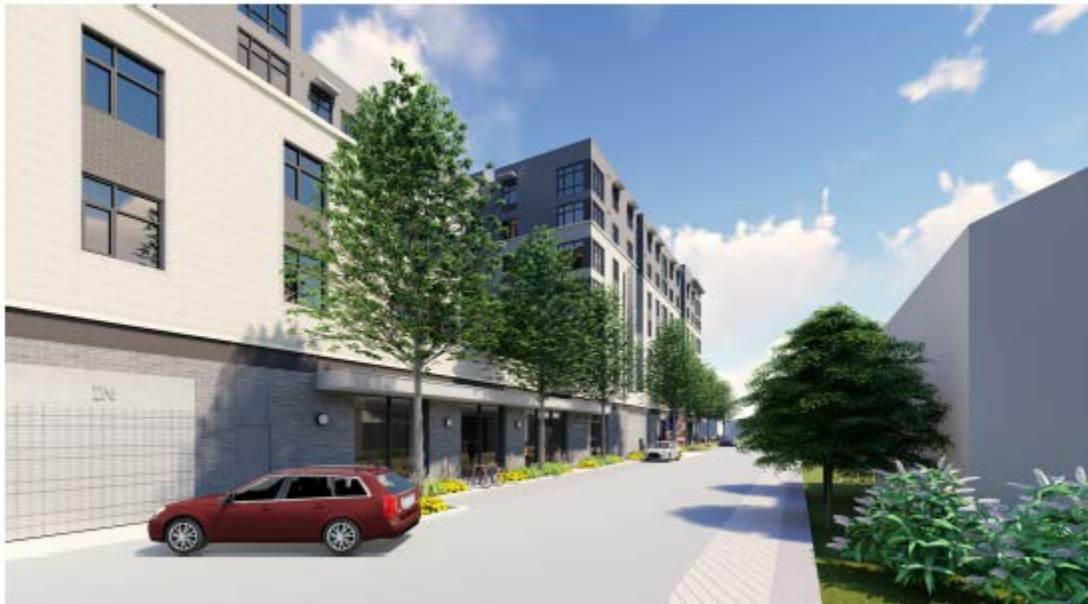
Figure 3—View from Northwest along new North/south connection
