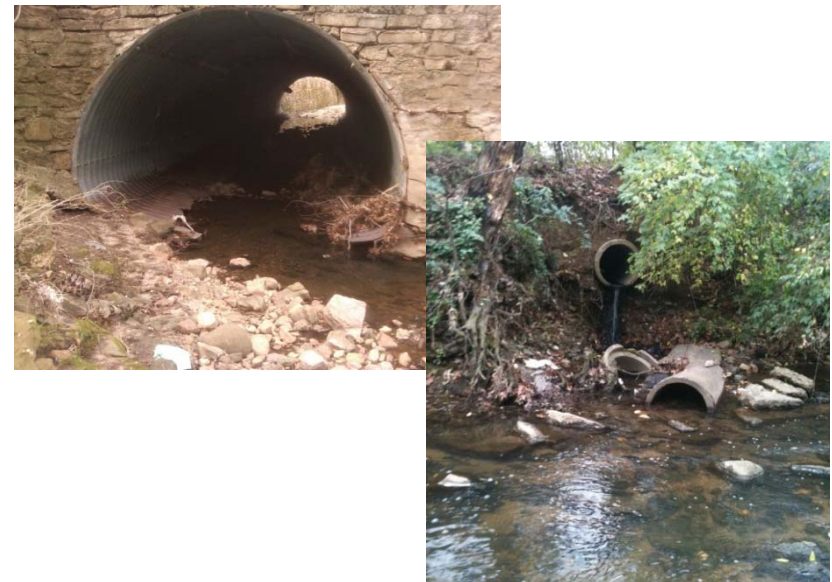
Capital Maintenance - $12.8 M
