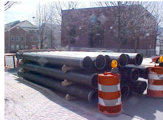
Water Distribution - $24 M
