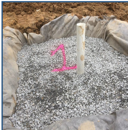
Photo of #57 stone installed
