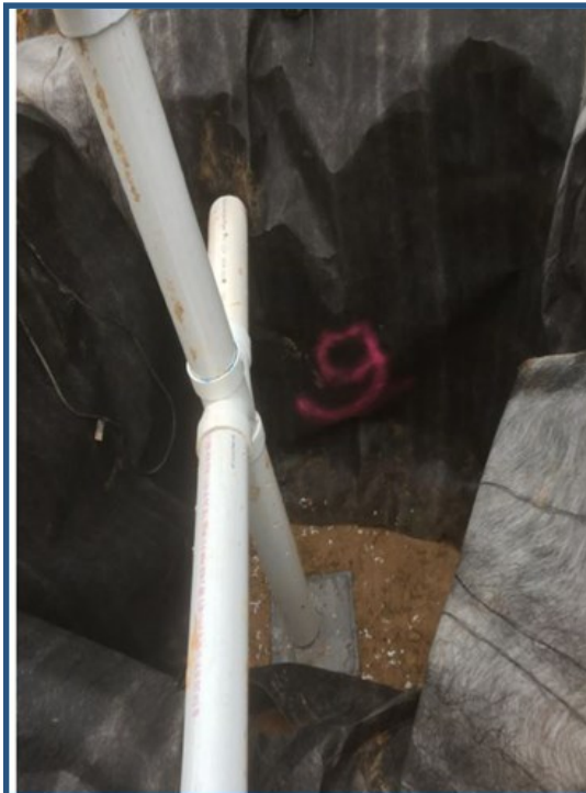
Fabric installed and perforated pipe installed.
