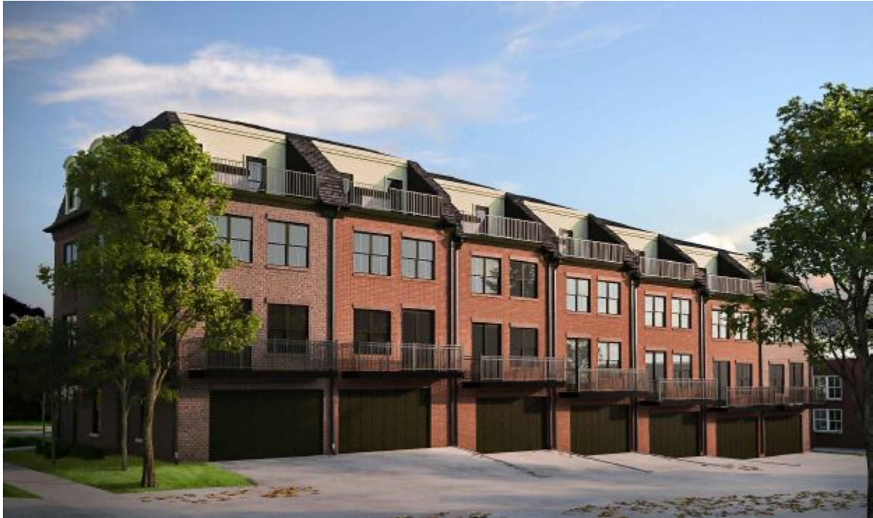
Figure 4: Building Architecture – view looking north from 12th Street South
